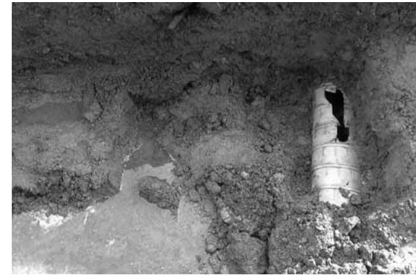
Fig. 2 - No Standing Water Around Pipe
